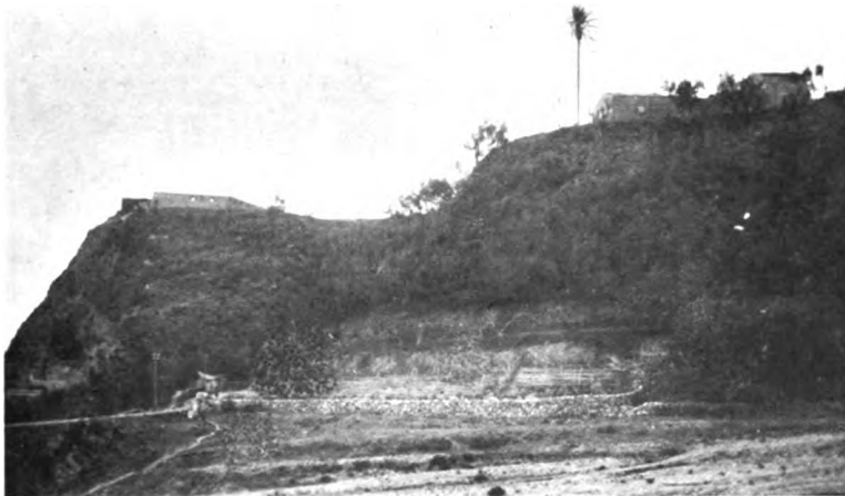
ALTIFIUMARA FORT (NOW 'FORTINO GARIBALDI').
